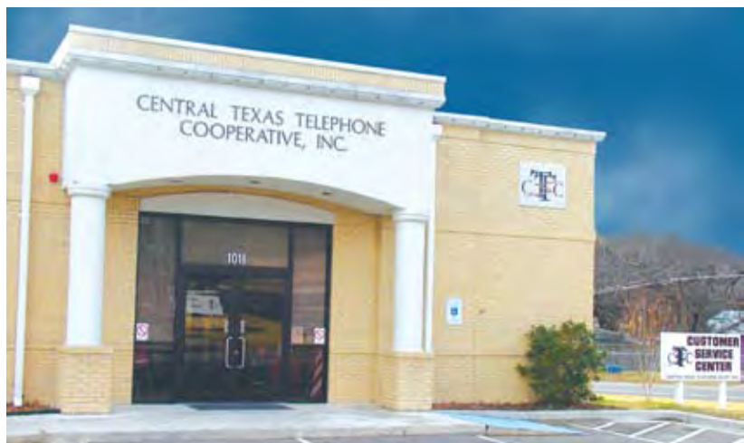
CTTC Customer Care Center in Goldthwaite, TX
