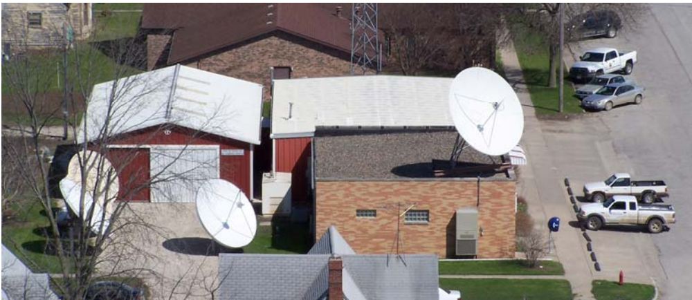
Stratford Mutual Telephone Company Facilities
